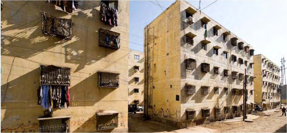
Picture 1: Labor square buildings
