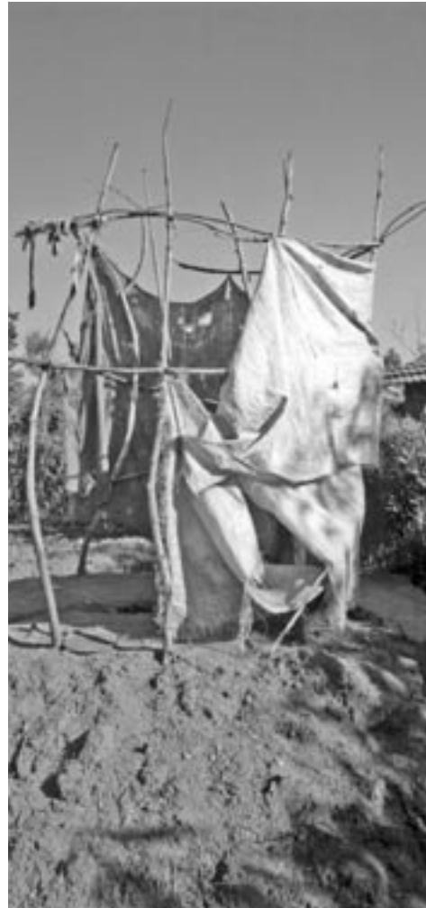
An unimproved pit-latrine in Nkwazi informal settlement, Ndola, Zambia
