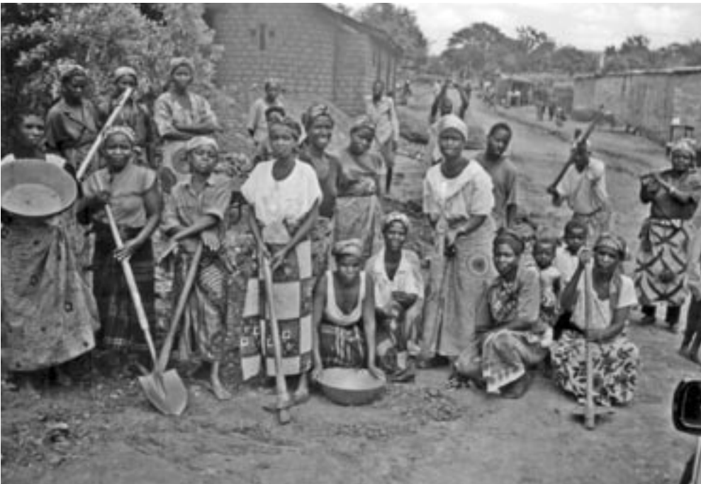
Residents of McKenzie making roads and storm water drains
