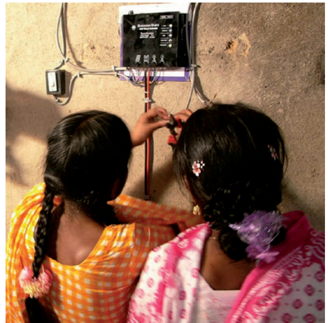
A woman technician installing charge controllers, Bangladesh. Credit: Grameen Shakti
