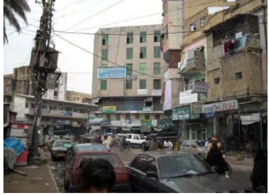
Jumbled overhead wires and kunda systems can be seen everywhere
